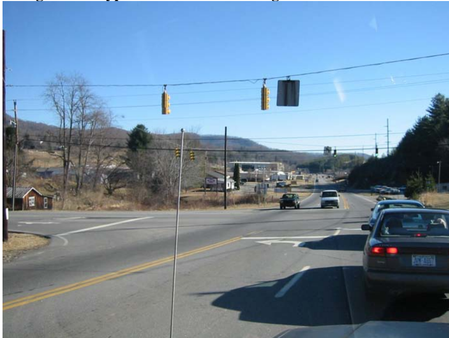
Figure 4 – Typical Intersection Along US-19 E in Burnsville
